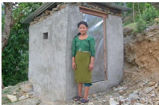
Newly rebuilt latrine
